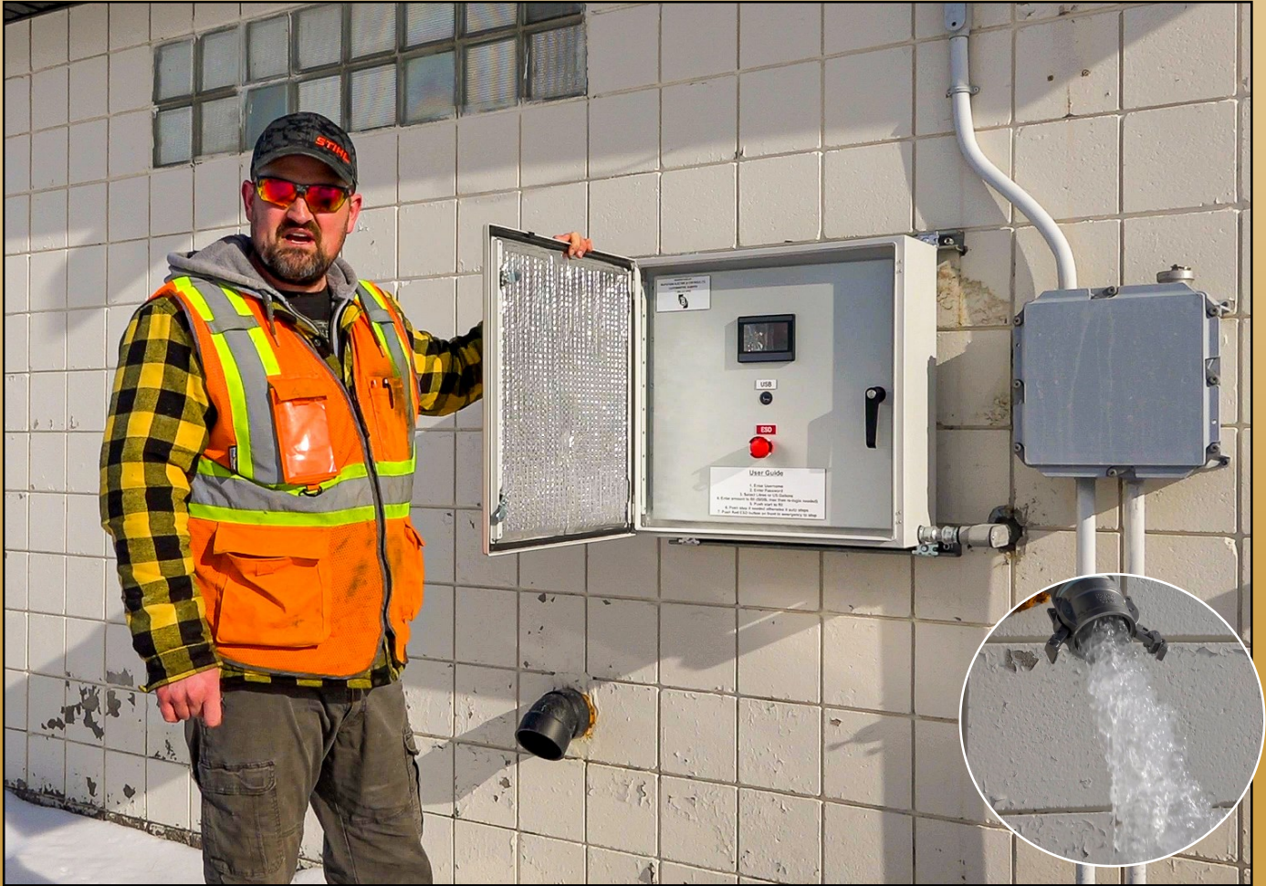
Hamlet Utility Operator Michael Northey displays the water sales panel at the Bulk Water Station in Strome. Inset: The hose is fitted with a camlock.
