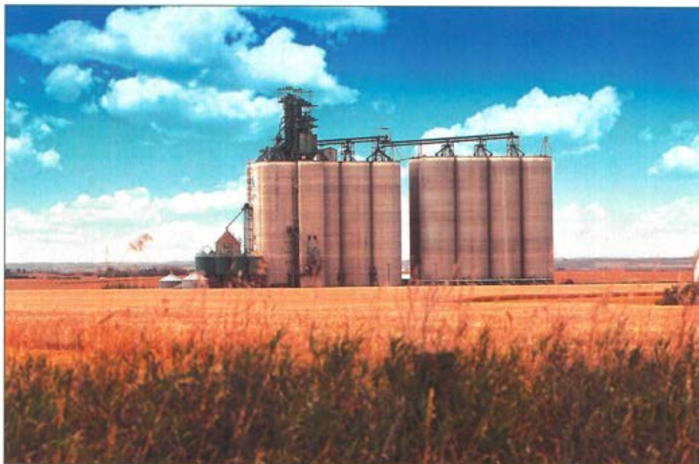
FIGURE 12: Viterra Inc. Grain Elevator in Flagstaff County Source: Flagstaff County
