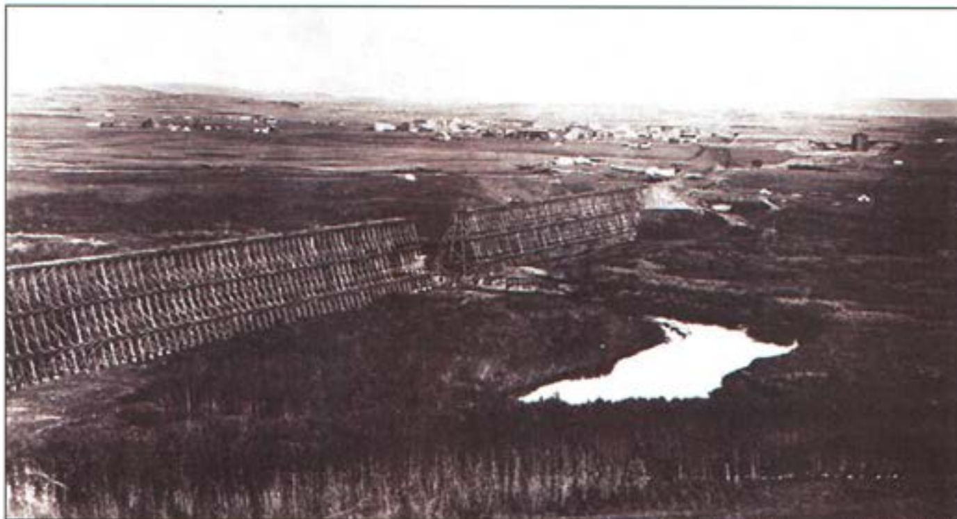
FIGURE 2: Construction of Bridge near Hardisty (1907) Source: Alberta Culture and Tourism
