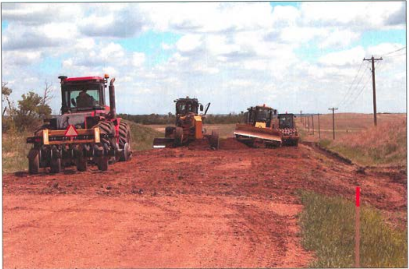
FIGURE 20: Road Maintenance Source: Flagstaff County
