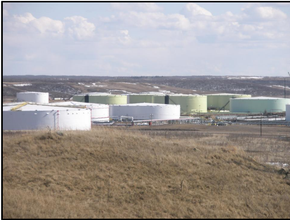
Figure 25. A Few of the Tanks at the Hardisty Hub
